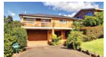
In most areas the largest residential developments took place in the 1970s and 1980s, so there is a mixture of original condition brick and tile.
